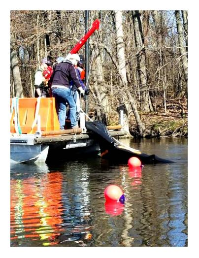
A 25-foot section of inland underwater oil barrier is laid out on a dock prior to deployment, April 23, 2018, in Kalamazoo, Michigan. The threefoot-high barrier is made of PVC and X-Tex fabric, and is designed to let water flow through while trapping oil. Weighted chains and scour flaps prevent oil and sediment from flowing underneath the barrier.
